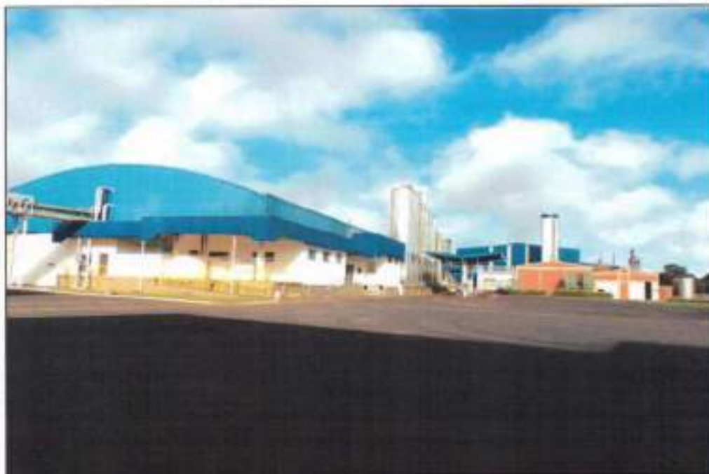
Vista externa – Complexo industrial – Cerqueira Cesar/SP
